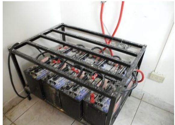
A battery Back-Up system for the server and communication equipment.
