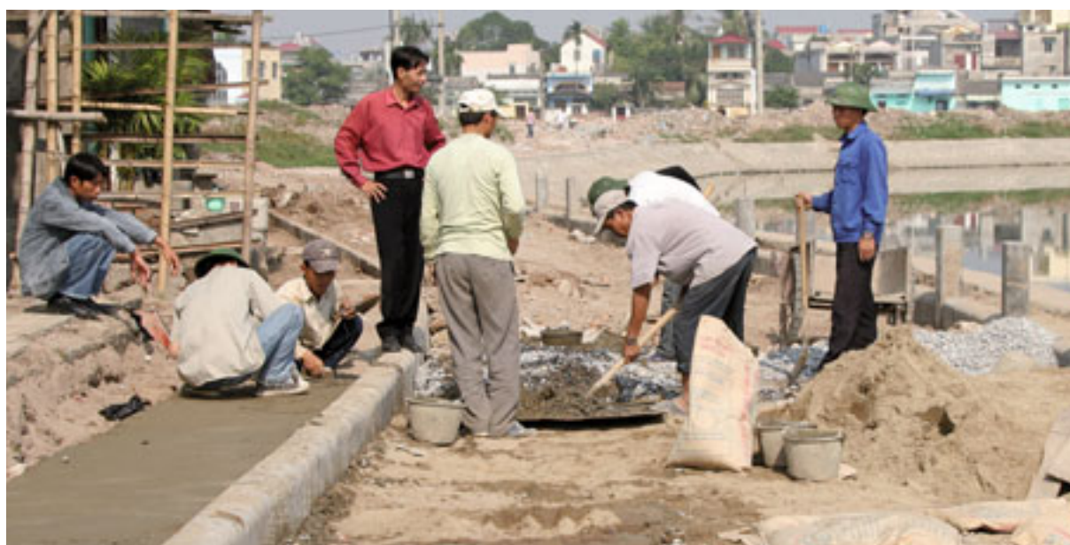
Constructing a water supply system in Haiphong. Photo: Jari Tenhunen
